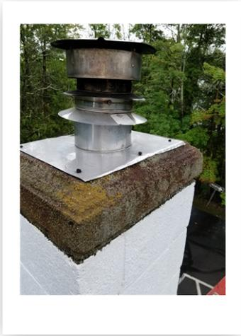
"The flue is covered with a cap but the rest of the top is not properly protected "
